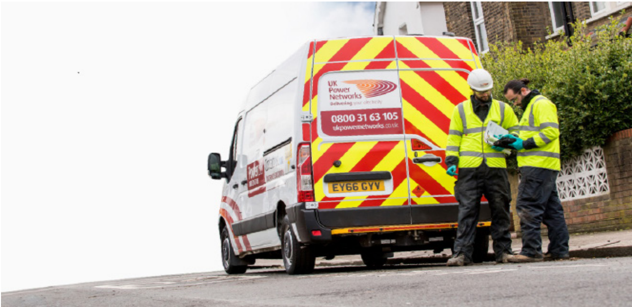
Photo ©UK Power Networks
